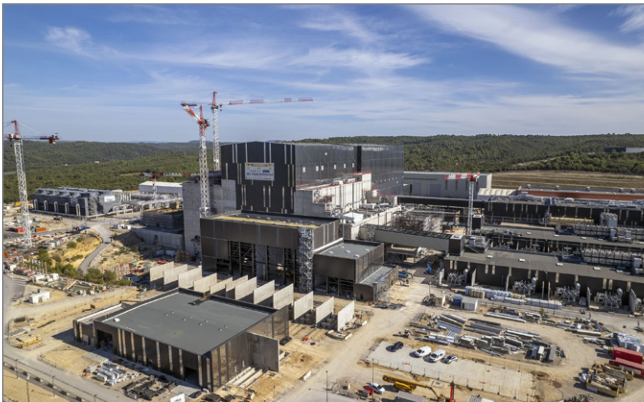
Figure 6: The ITER site in September 2023, showing the tokamak building.
