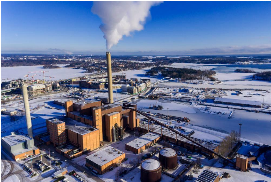
Figure 6: The Hanasaari power station.
